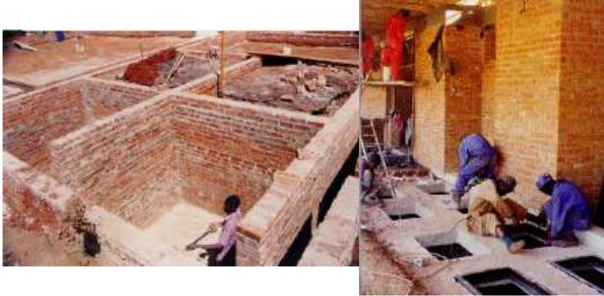
Figure 4.4: Rock-store compartments during construction of the Middle School
