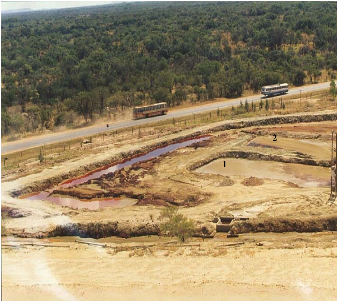
Figure 2.7 Shows what was once two separate storage ponds 1 and 2, the deep red water is an indication of iron ( \text{Fe}^{3+} ). The vegetation on the top left side of photograph across the main road shows no sign of effects from the acidic waters from the dam while the vegetation close to the dump has been affected. Buses for scale.
