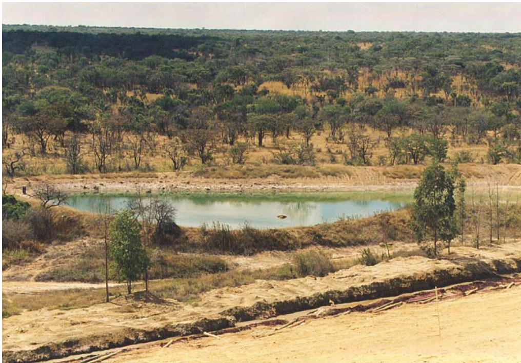
Figure 3.2 A storage pond at Athens mine. Note the green colour of the water due to copper, and the white salt deposits on the sides.
