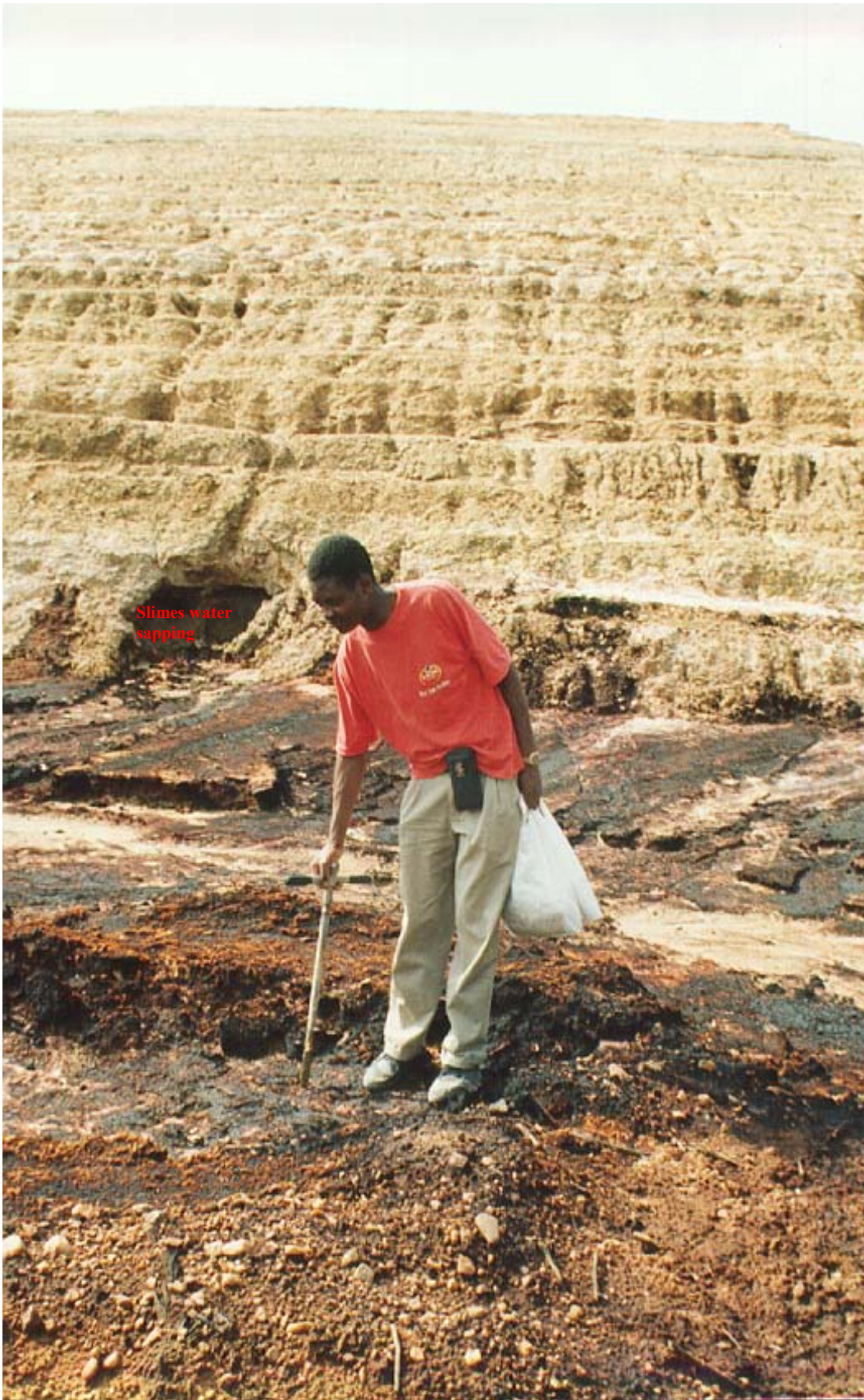
Figure 2.10 The slimes dam with compacted layers and the crystals at the base with the gullies from run off water on the surface of the dump and slimes water sapping at the base of the dump.
