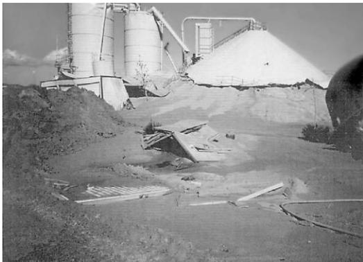
Figure 1: A 9 000ton silo split apart about two weeks after it was first filled to full capacity
