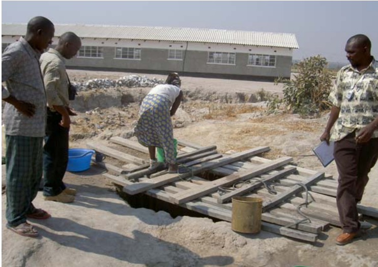
Figure 3: A communal well at Kawama Primary School used for domestic purposes
