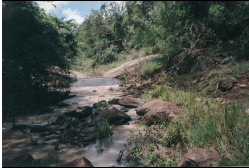
Figure 5.3: Trapezoidal flume used to measure runoff from Romwe catchment.
