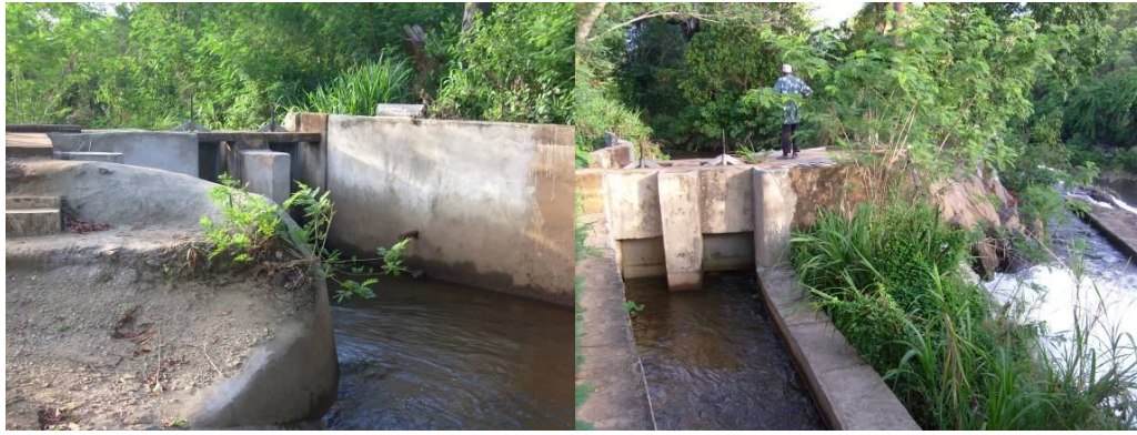
Figure 3.5 The intake structures of the Mkindo Irrigation Scheme
