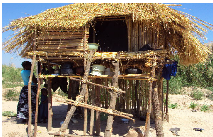
Figure 4. 18: Elevating hut, coping with floods
