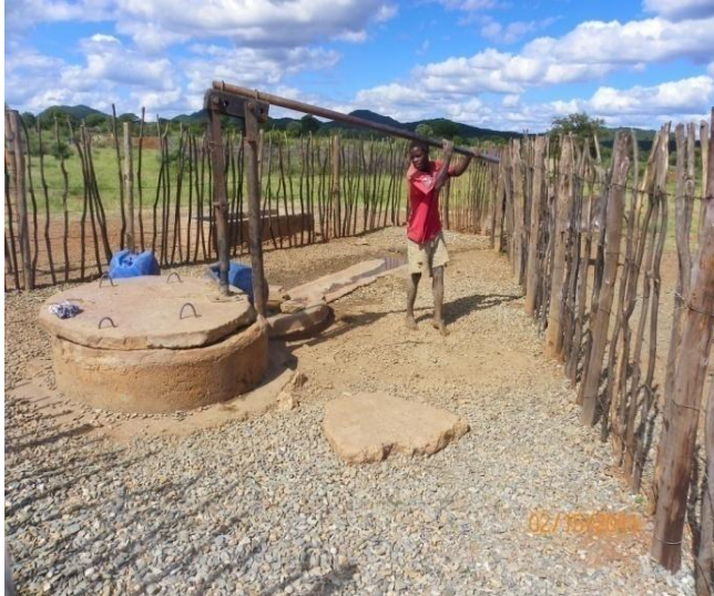
(a) Nyelane Well in Ward 1 fitted with bush pump
