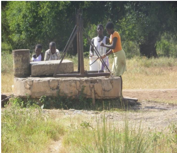
(e) Mpasikwe Well) in Ward 2 with windlass and bucket system
