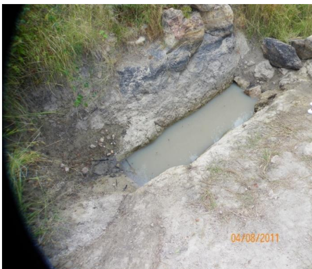
(g) Unprotected shallow well in Thuthuka Village, Ward 1
