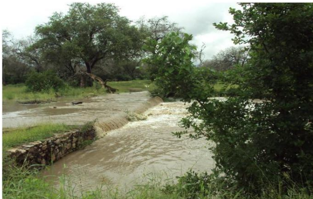
Figure 3. 3: Mana River flowing over the bridge to Nyamepi camp
