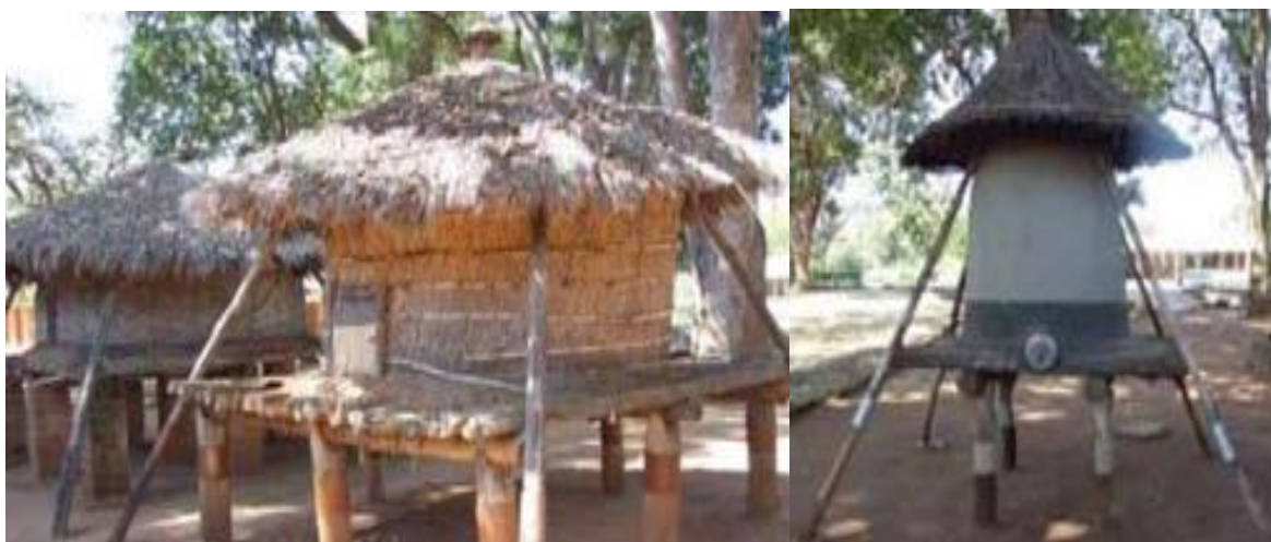
Figure 4.6: Two traditional outdoor woven granaries constructed from grass or bamboo for storage of cob maize or groundnuts (left), granary with mud-plastered walls for storage of shelled maize grain (right). Note; the base elevation and the rat guards are not the typical traditional ones with conical shape. (Source: Charles Singano, the Department of Agricultural Research Services, Lilongwe, Malawi).
