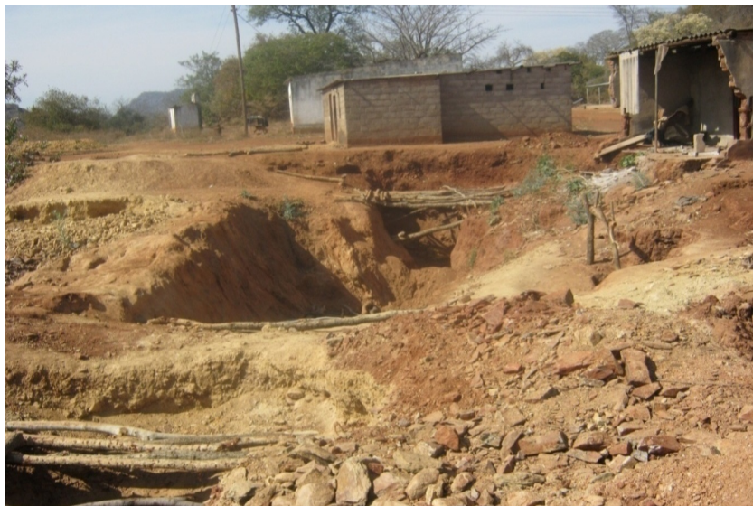
Plate 4: Destruction of Infrastructure due to mining. Source: M. Jomboro, 2018.
