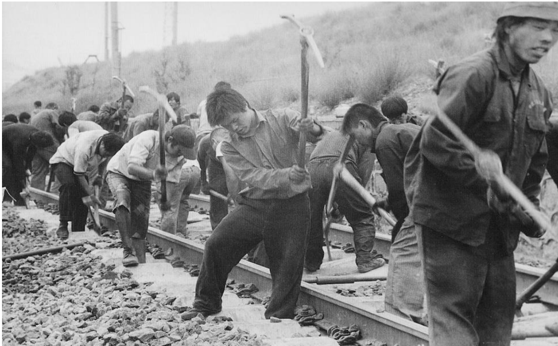
Fig 1: Neglect of OHS on Railway Slave Work
