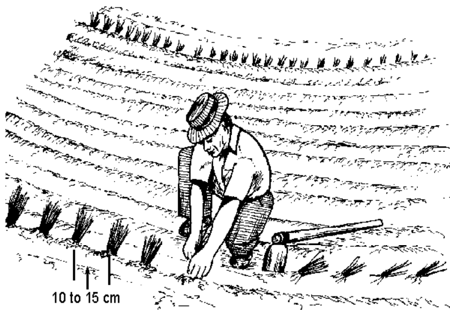
Figure 52 Planting a Vetiver Grass hedge in front of a drain
