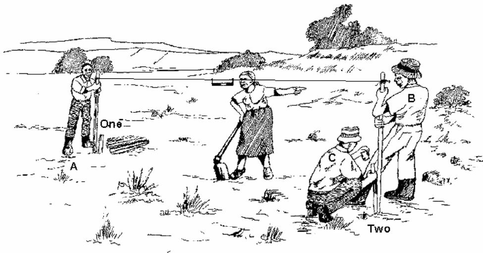
Figure 27 Step 4 - line level
