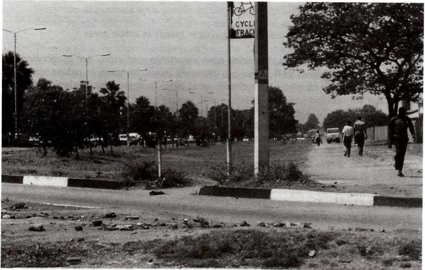
Fig.16: A poorly maintained cycle track with no lights.
