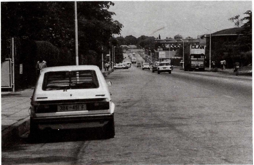
Fig.1: A major road leading into an industrial area in Harare.
