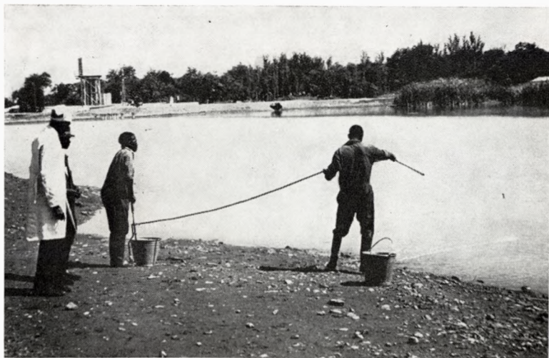
Fig. 25. Use of stirrup pump to apply molluscicide for local control of snails.
