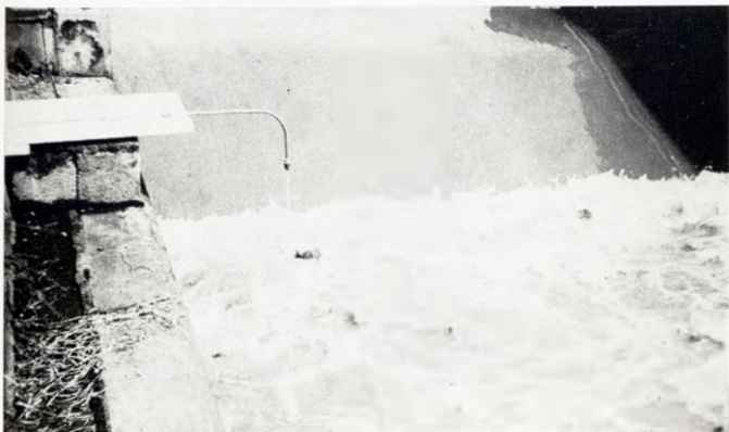
Fig. 23. Application of molluscicide to main irrigation supply canal of a sugar estate, using a simple constant-flow device.
