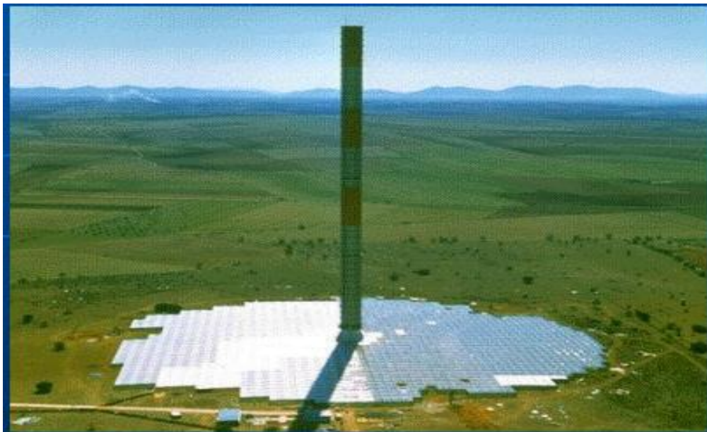
Figure 3: Solar chimney power plant at Manzanares, Spain
