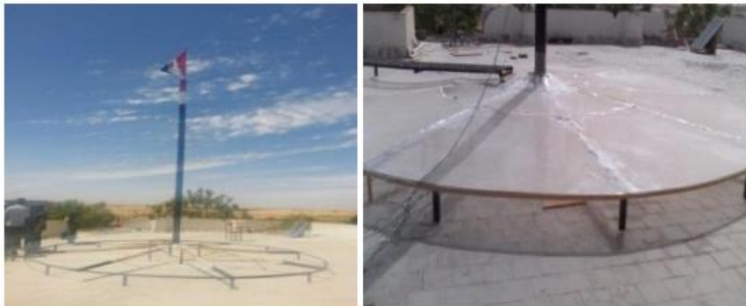
Figure 4: Small scale solar chimney plant prototype
