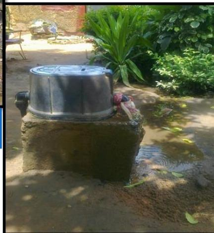
Leakage on the connection line connecting the water meter in Zambezi Sawmills
