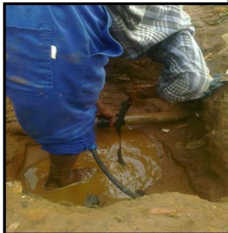
Using improper fitting for sealing a leakage on a 50 mm AC pipe in Villa Estate
