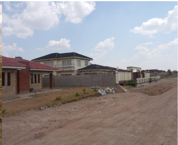
Figure 6: Residential location under construction on previously fields
