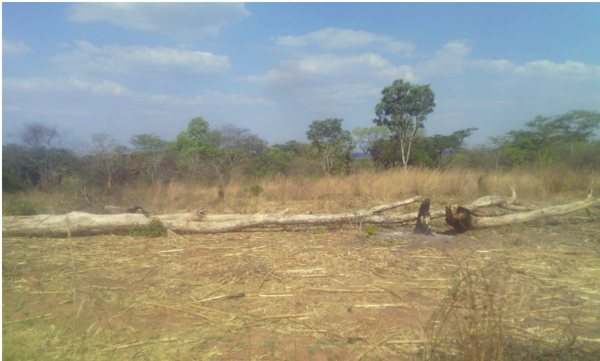
Figure 8: Land clearance in progress
