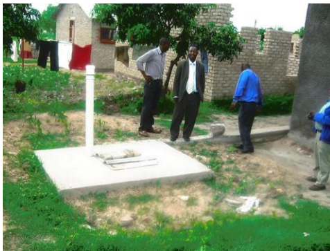
Figure 4.5 Septic tank in a high density area of Chitungwiza ( less than 1,000 m 2 stand size).
