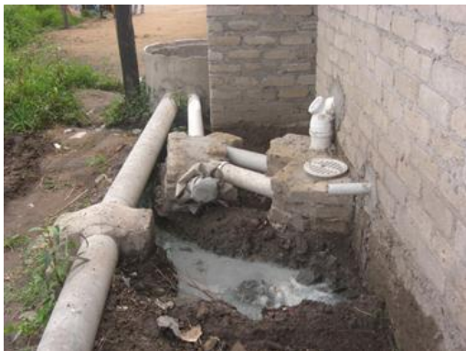
Figure 4.11 Poor workmanship in sewer connections can cause silt to enter and block sewerage network systems
