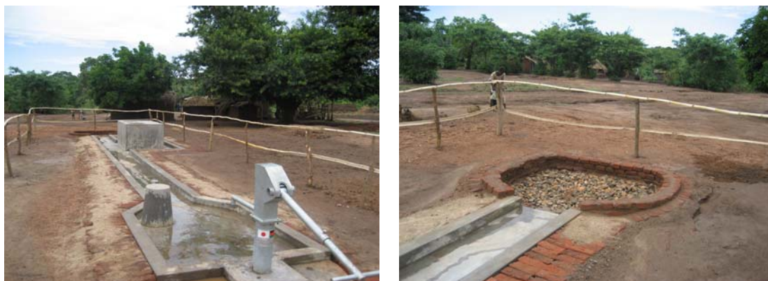
Photo 5.2: High yielding (3.3L/s) borehole at Nabvumi village (Kamanzi Dam)
