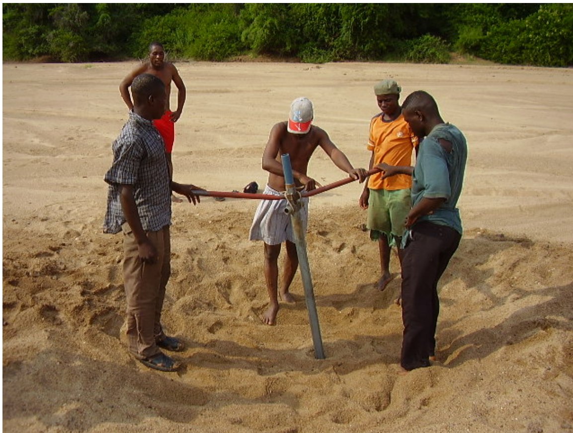
Fig 4.3.1 Manual technique for the Installation of piezometers
