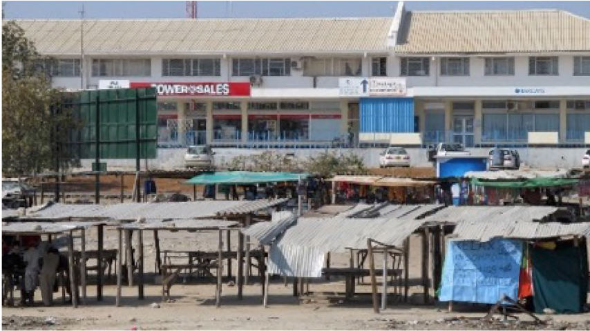
Plate 1: The relationship between the informal structures and Block A
