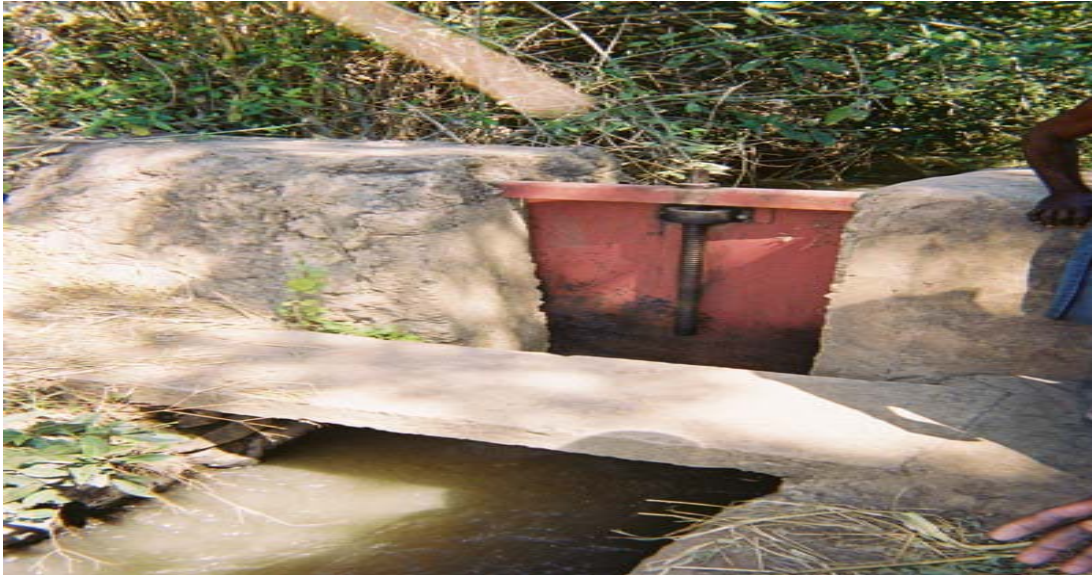
Plate 1: Concrete irrigation canal
